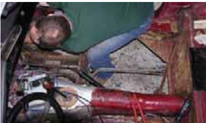
8. After removing as much as possible with the body saw, we attacked the spot welds with an air chisel. We put the chisel between the remaining floor pan sheetmetal and the body sheetmetal. (Be careful not to cut the latter.)
