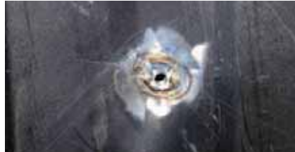
11. Because of crossbrace interference, the seat nuts must be welded onto the new repro pan before it can be installed.
