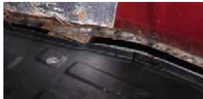
12. On the replica pans, we trimmed away most of the vertical sheet metal. We left it only where we had rust-throughs on the body.
