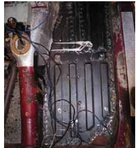
17. After the pans were welded in, I sprayed their bottoms with undercoat, applying two coats at the seams. After a coat of primer was dry, I caulked the inside seams with a good butyl rubber caulk. (Do not use silicone caulk, which can release acetic acid as it dries.) I then used a high-quality primer on the interior surfaces of the pans and any bare metal.
