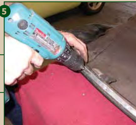
5 We drilled out the rivets using an 1/8-inch drill bit in a cordless drill.
